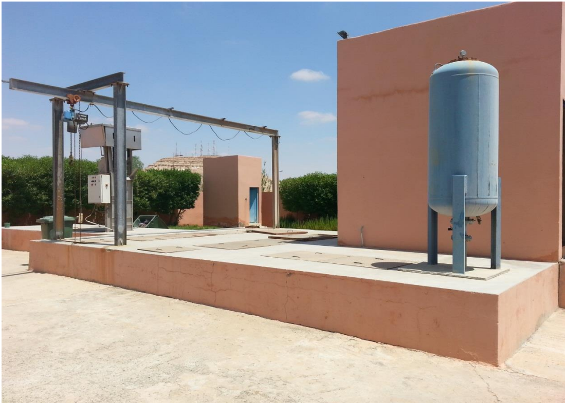
Fig. 12: station de pompage
