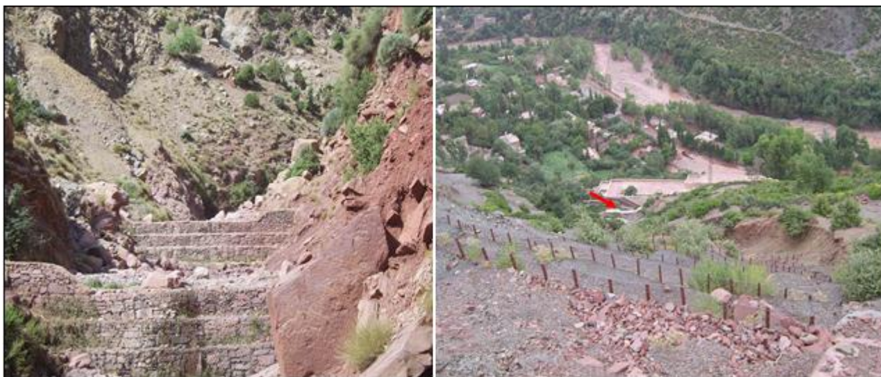
Figure 17: seuils en gabion (DREF, 2010)
