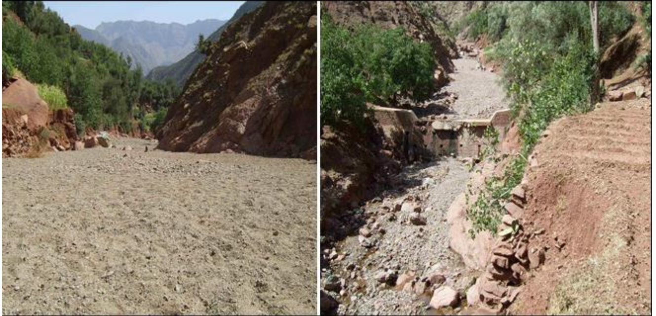
Figure 19: correction de pentes (DREF,2010)
