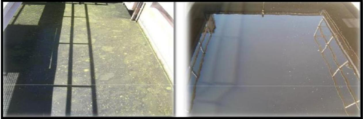
**Figure 10. Bassins de coagulation-floculation**
