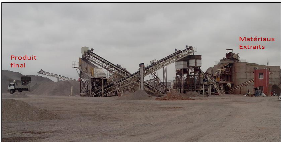
Figure 11: station de traitement.
