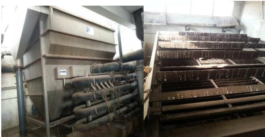
Figure 13: Flottateur existant [7]
