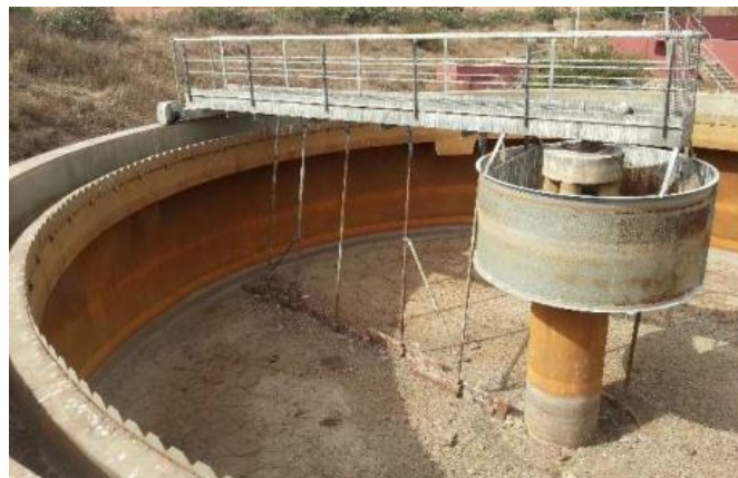
Figure 15: Clarificateur existant [7]
