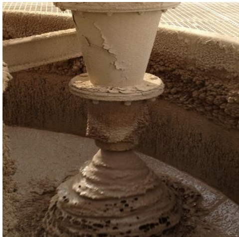
Photo 7: Hydrocyclone classificateur
