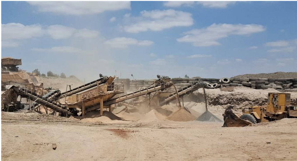
Figure 18 : Station de remblayage
