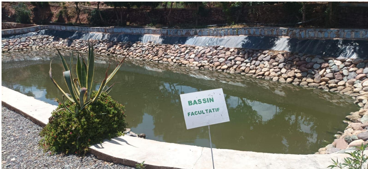
Figure 19 : bassin de maturation (Asselda)
