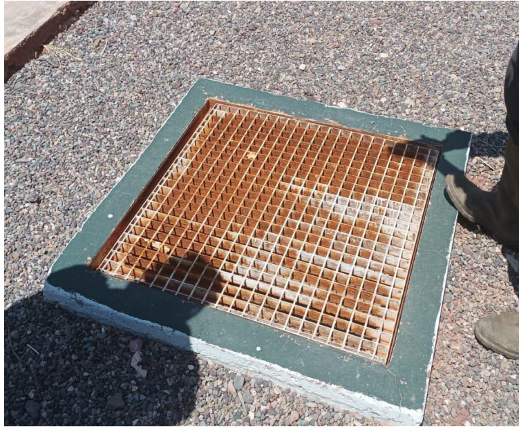
Figure 17 : Regard de communication
